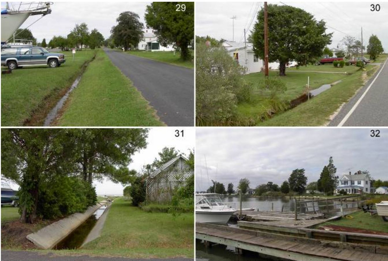
Photos 29–32. Lewisetta, Virginia. Photos 29 and 30 show tidal ditches along the streets of Lewisetta. The concrete-lined ditch in the foreground of Photo 31 conveys water from a ditch along the street to the Potomac River. In the background is a seawall along the Potomac, and a tide gate, which allows the ditch to drain except during high tides. Photo 32 shows low, but somewhat higher, development behind bulkheads along the protected shore on the east side of the community. October 12, 2002.
