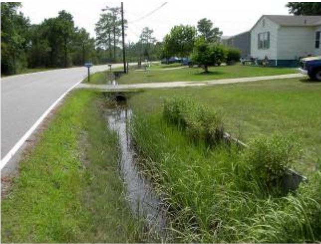
Photos 11–12. Tidal Ditches in Poquoson. Photo 11 shows wetland vegetation in a tidal ditch. Photo 12 shows a wooden bulkhead along the shore of a tidal ditch, to prevent a front yard from eroding into the ditch and blocking drainage (October 2002).
