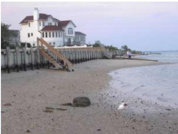
**Photos 30 to 32. Shore protection structures can block the inland migration of mudflats, vegetated wetlands, and estuarine beaches.** Top: a retaining wall along tidal flats in Westchester County, New York (March 2003). Middle: a bulkhead along a tidal marsh in Monmouth, New Jersey (September 2003). Bottom: a bulkhead along South Jamesport Beach in Riverhead, New York (September 2006). Photo source: ©James G. Titus, used by permission.
