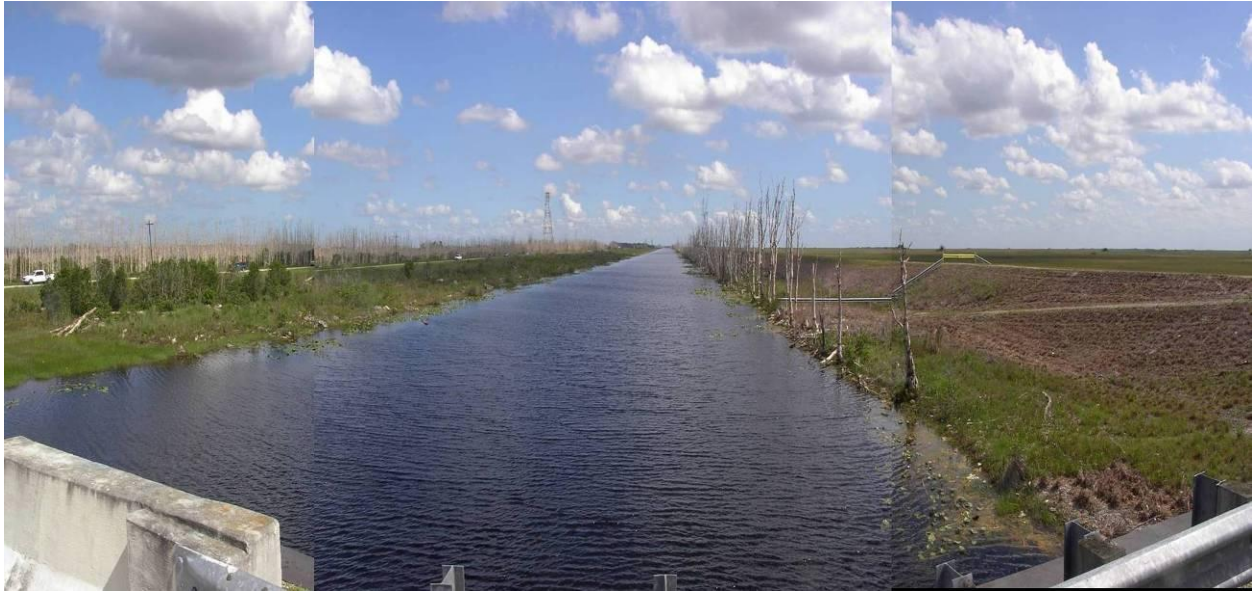
Photo 4. Levee Along Krome Avenue (June 2005)
