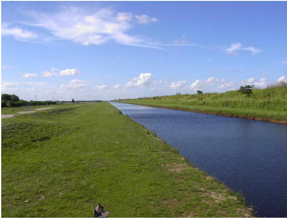
Photo 5. Canal and levee with agricultural lands to the west. This photo is near the Howard Drive crossing of the levee, into the largest agricultural area outside of the levee system. June 2005.
