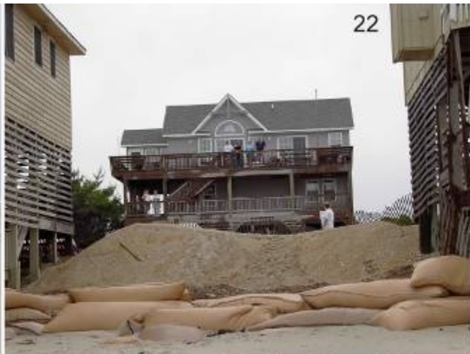
Photos 21–22. Geotextile containers protecting homes along the shore at Nags Head (June 2003).
