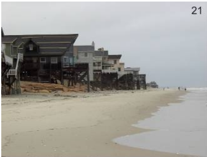
Photos 21–22. Geotextile containers protecting homes along the shore at Nags Head (June 2003).
