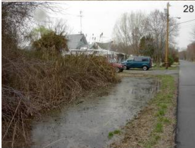
Photos 26–29. The Gibbstown Levee. The water behind the levee to the left appears to be a few meters lower than the Delaware River (26). The Commodore Barry Bridge is in the background. Because drainage is determined by a tide gate (Photo 27), the water levels will be no lower than the low tide level, leaving the lands behind the dike (Photos 28–29) vulnerable to flooding as sea level rises. These areas are already below sea level (March 2003).
