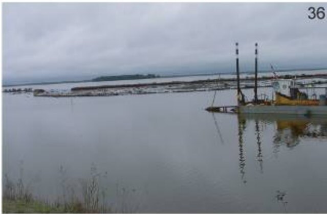
Photos 34–37. Blackwater Wildlife Refuge. (34) Waterfowl amidst deteriorating marsh. (35) Water control structure to prevent saltwater intrusion and marsh drowning. (36) A dredge restorer eroded marsh by moving material from newly formed shallow waters to (37) areas marked for marsh creation (October 2002).
